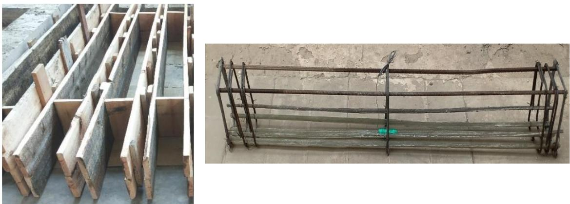
Fig. 4. Details of Reinforcement and Wooden Forms.
